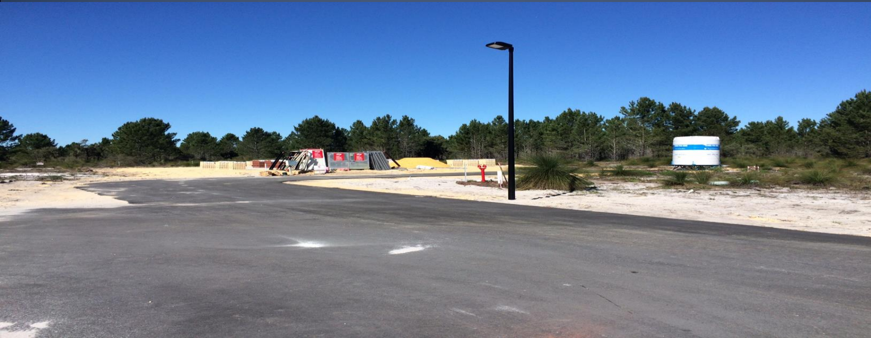
Caretaker cottage under construction
